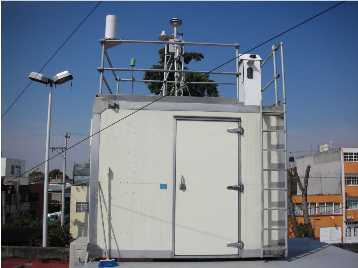
Figure 3-2. Photo of SS1 Site on the Roof of the SIMAT Laboratory Facility
