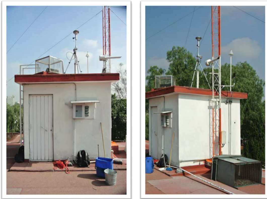
Figure 3-6. Front and Side Views of the PED Site Shelter
