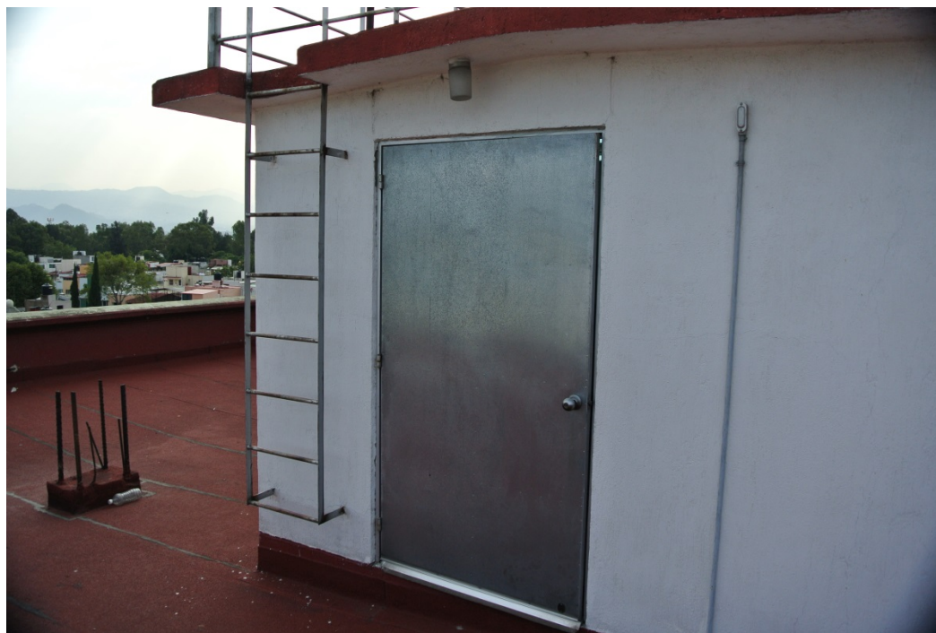
Figure 3-7. Front View of UAX Shelter
