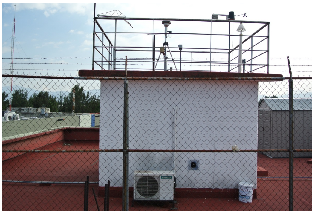
Figure 3-8. Side View of UAX Shelter
